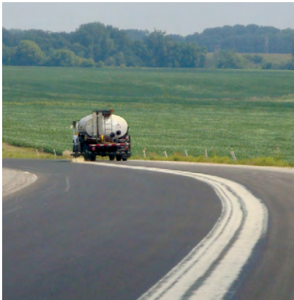
JOINTBOND Being Applied to Longitudinal Joint Area
